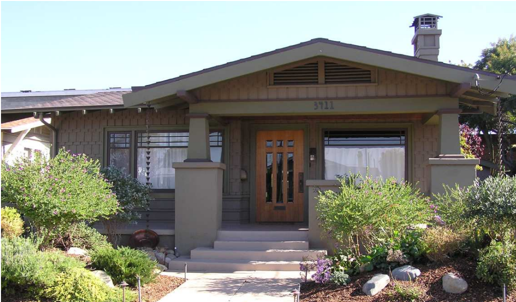
Eldora Rudrauff House, 3411 29 th Street, Resource #558 Photo Courtesy of Katherine Hon, December 27, 2008
