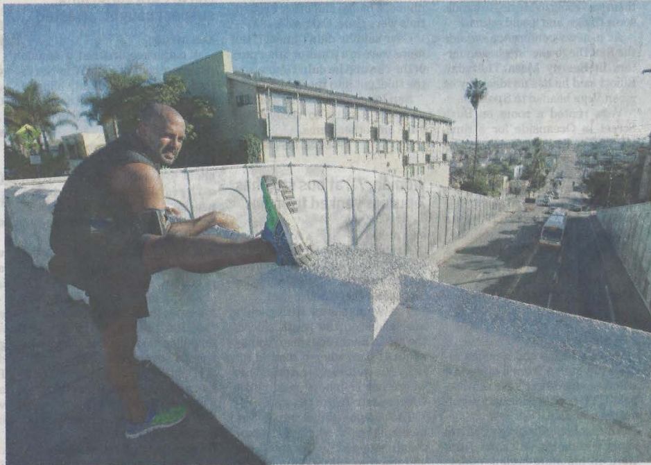
Anthony Romero stretches on the Georgia Street Bridge, overlooking University Avenue, recently. The 1914 bridge will be restored with a fresh look and earthquake-safe construction. JOHN GASTALDO • U-T
