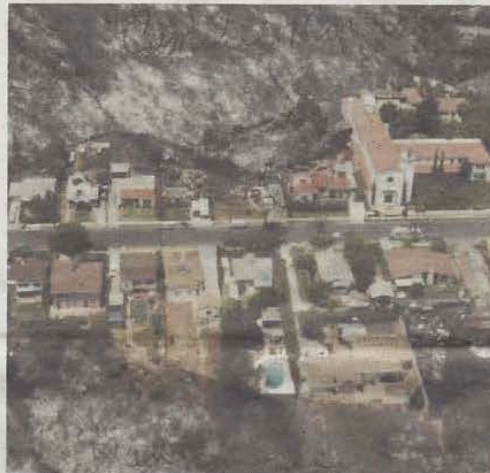
The fire damaged parts of the Carmelite Monastery on Hawley Boulevard but spared the main buildings, upper right. (Photo by Bob Stemen)
