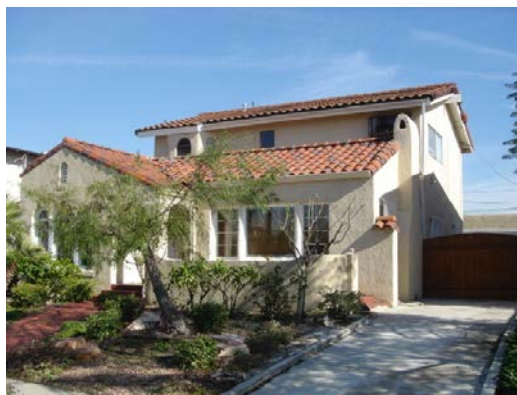
HRB Site # 1008-012 – North Park Dryden District Contributor, 3511 28th Street built in 1925 in the Spanish Colonial Revival Style
