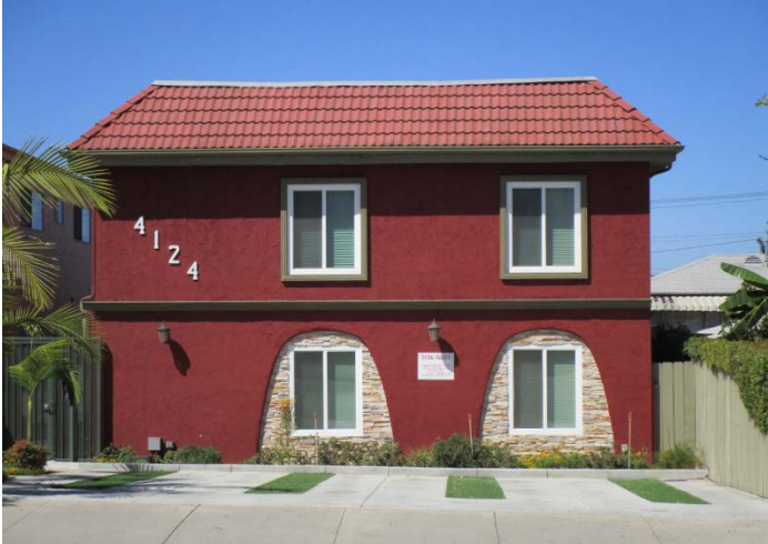
Two-story, 7-unit Huffman at 4124 Texas Street.
