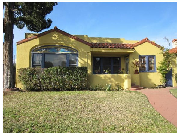
3530 Mississippi Street built by Master Builder John Pearson
