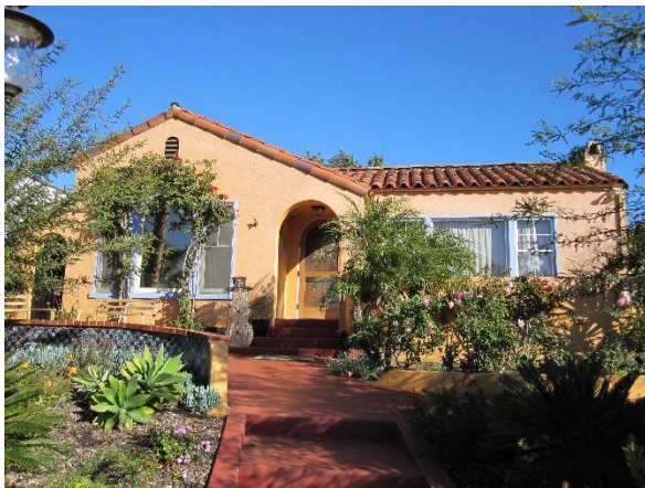
3435 Texas Street, Designated Built by Master Builder John Pearson
