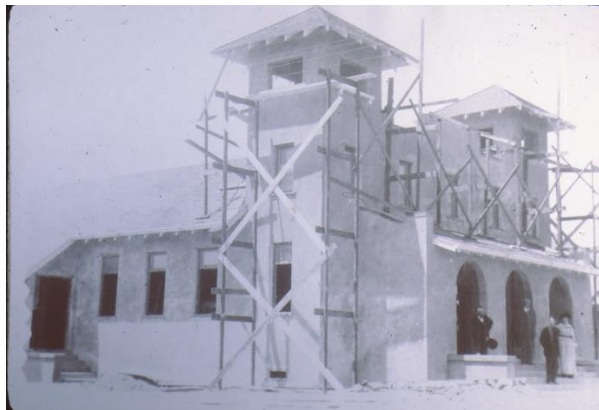
Under construction in 1914
