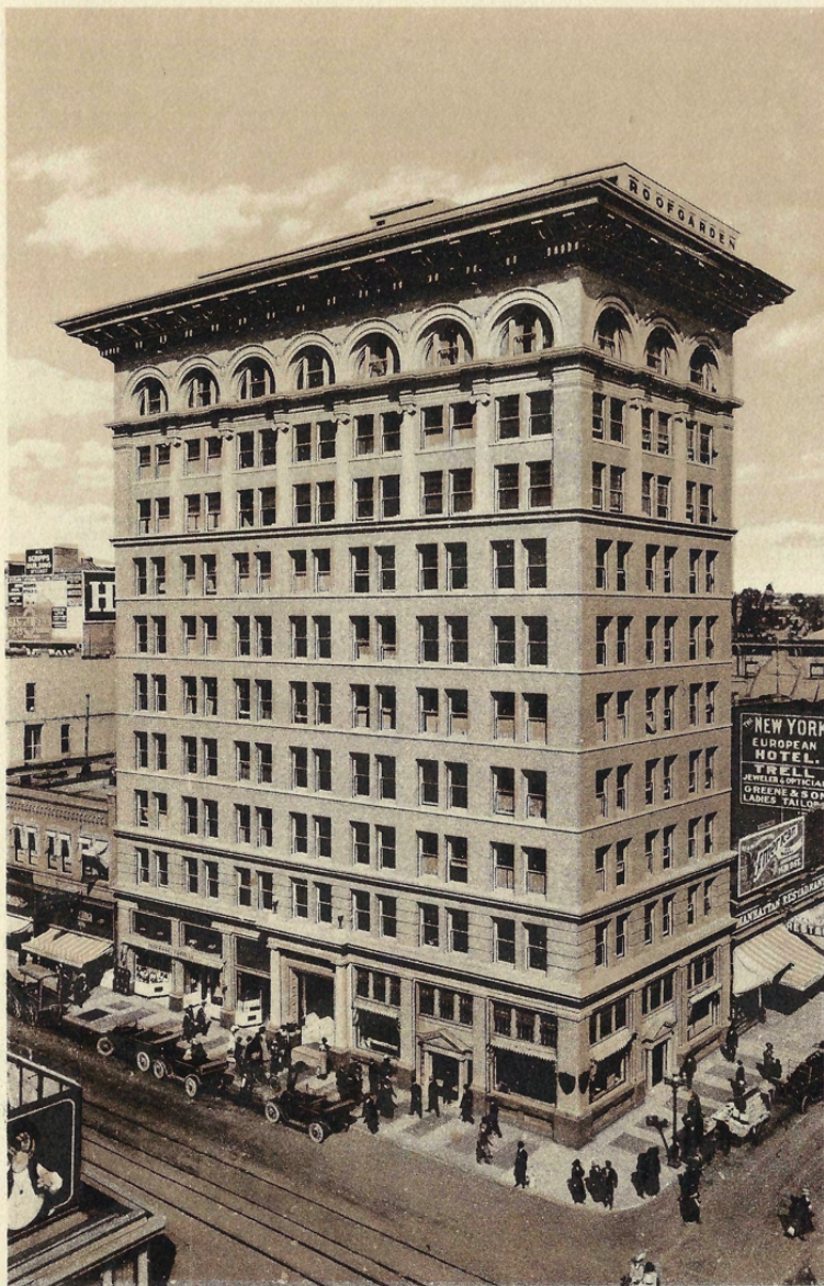
American National Bank Building.
