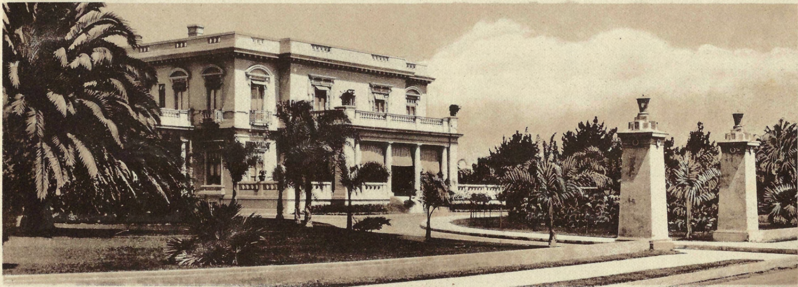
Residence of John D. Spreckels, Coronado, San Diego.
