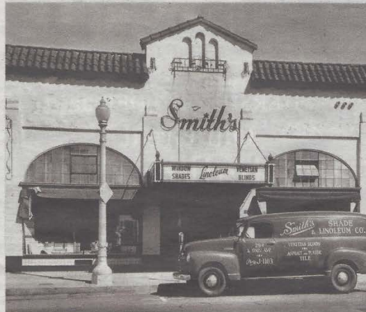
This undated photograph is from the decades when Smith's Shade & Linoleum anchored the eastern space of the Newman/I.O.O.F. building. (Courtesy of North Park Historical Society)
