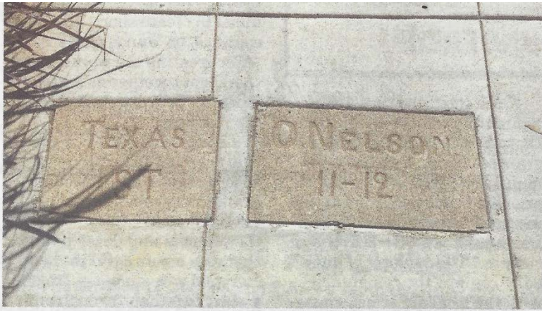
Present-day contractors must save and reset historical street name and contractor stamps. This relocated stamp for Olaf Nelson dated November 1912 is at the northwest corner of Texas Street and Myrtle Avenue.
